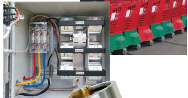
Figure 2: A Rayvoss “A” system, that included Strikesorb 80s, a light-emitting diode (LED) indicator and surge counter was installed, after the generator changeover switch to regulate both utility surges and surges coming from the generator.
