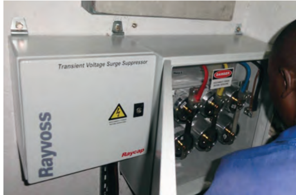
Figure 3: SPAR interior installation of the Rayvoss system.
