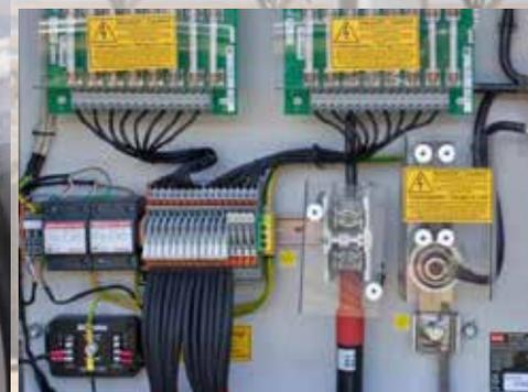
*Strikesorb 35 designed for photovoltaic DC power circuits.*
