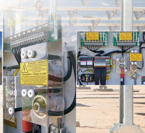
Strikesorb 35 designed for photovoltaic DC power circuits.
