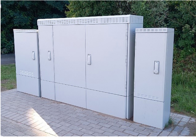
All aluminum Raycap NVT & MFG cabinets in the field, quite a contrast between aluminum and polycarbonate.
