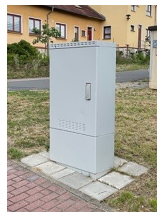
Aluminum enclosures have many advantages such as resistance to weather and ageing, high mechanical strength, easy cleaning and 100% recyclability.
