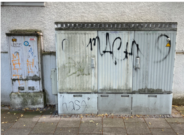
Polycarbonate cabinets get gray and dull with age, and cannot be easily cleaned or brought back to their original exterior look.
