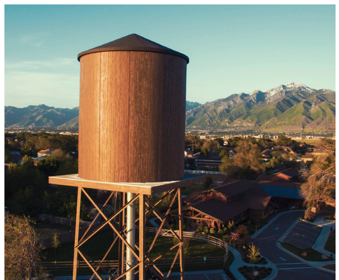
A macro cell site concealed within a water tower can provide 5G service across a non-urban location.
