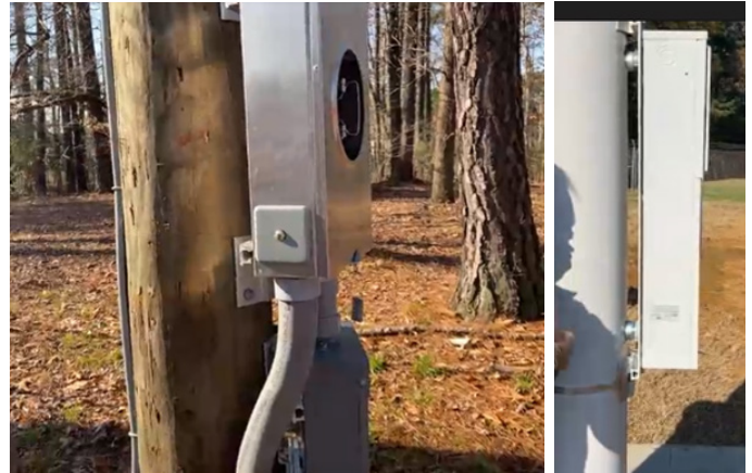
Figure 3: The Raycap Combination Meter/Disconnect unit replaces multiple boxes and their cabling with one sleek unit that looks good on wooden or steel poles.
