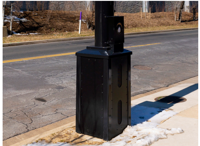
The square base design provides more room for equipment, and removable panels, than a circular one.
