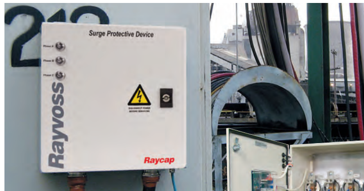
Rayvoss installed on a conveyor belt
