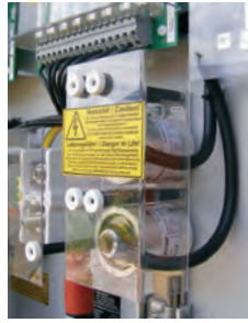
Figure 2: Junction box installation
