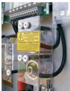
Figure 2: Junction box installation
