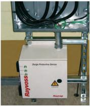
Figure 2: Rayvoss installation inside engine generator shelter.
