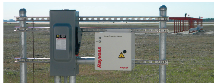
Figure 3: The Rayvoss Surge Protective Device (SPD) protects the incoming power for the localizer shelter.
