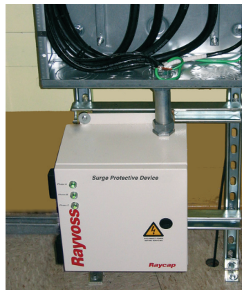
Figure 2: Rayvoss installation inside engine generator shelter.
