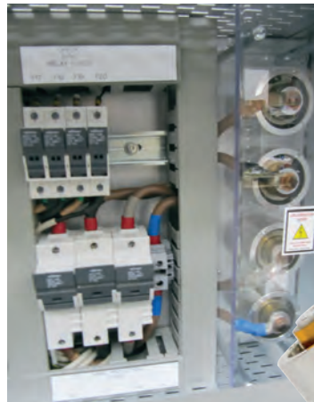
Figure 2: Strikesorb 40 modules integrated on a busbar inside a power distribution panel
