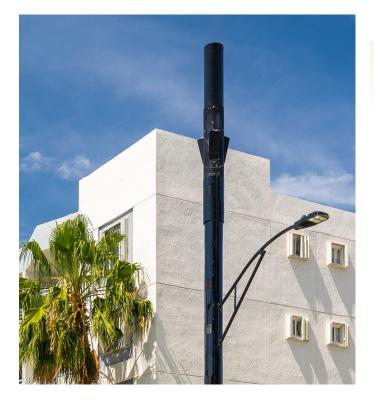
Another requirement concerned mounting the 5G radios at the top of the pole. The pole design tilts the radios between 15 and 20 degrees for better coverage at the ground level, a requirement that is becoming more common in our projects. It takes extra effort to design shrouding that goes between the radios to improve the aesthetics of the top of the pole. In the end, our team and the customer were happy with the results.
