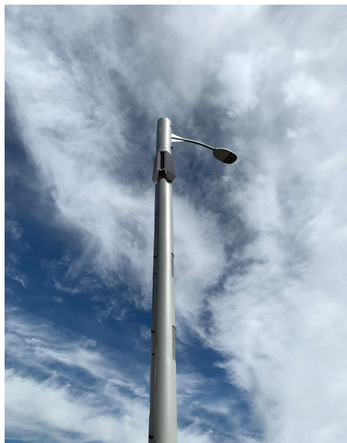
Raycap LA BSL demo pole with exposed 5G radios.
