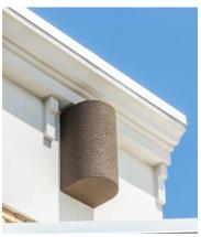
**Rooftop:** Ballasted (nonpenetrating) concealment pods disguise rooftop antennas using a steel frame, center mast pipe, steel clamp-on bulkheads and a radome. These standard frames allow for reduced engineering cost and lead time plus the optimized framing material simplifies manufacturing and installation.
