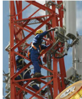
Figure 3: Installing a Raycap CM surge protection device adjacent to the RRH.
